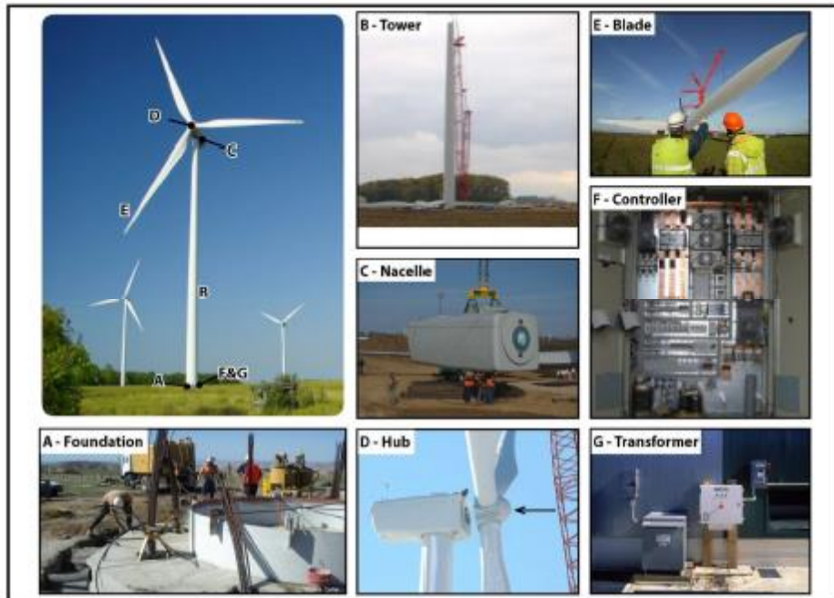
Figure 2-1 Wind Turbine Generator Components
