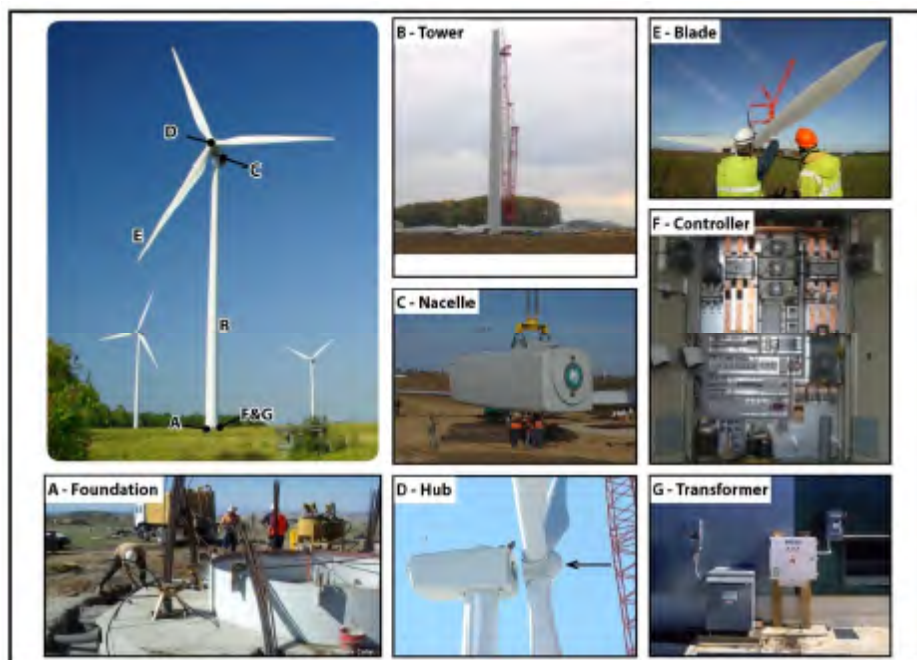
Figure 2-3 Wind Turbine Generator Components
