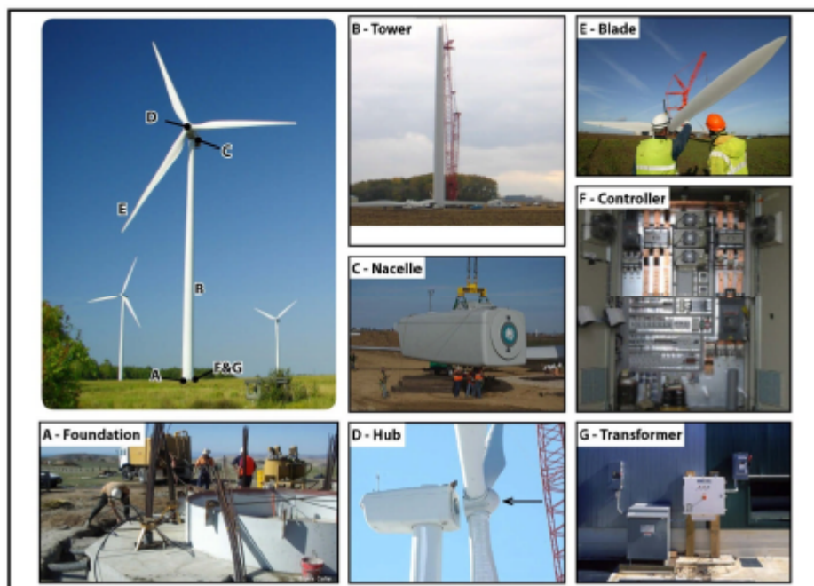
Figure 2-3 Wind Turbine Generator Components
